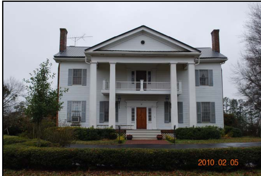
Figure 5: 2010 Photograph of Front (West) Facade
