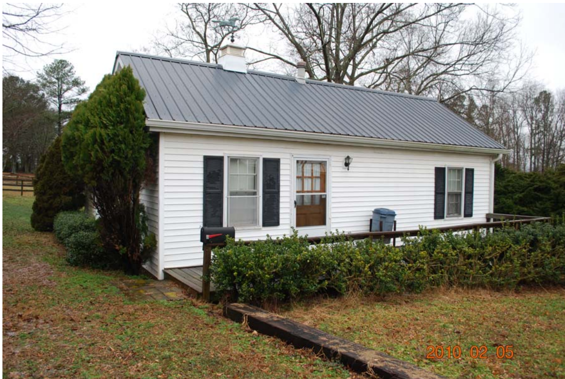
4A: Northwesterly View of Southeast Oblique of ECA Structure 4
