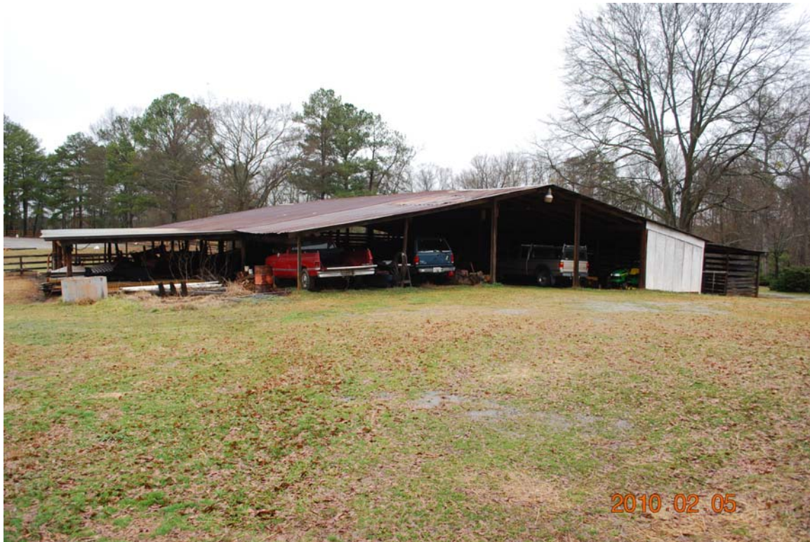
3A: Northwesterly View of Open Shed (ECA Structure 3)
