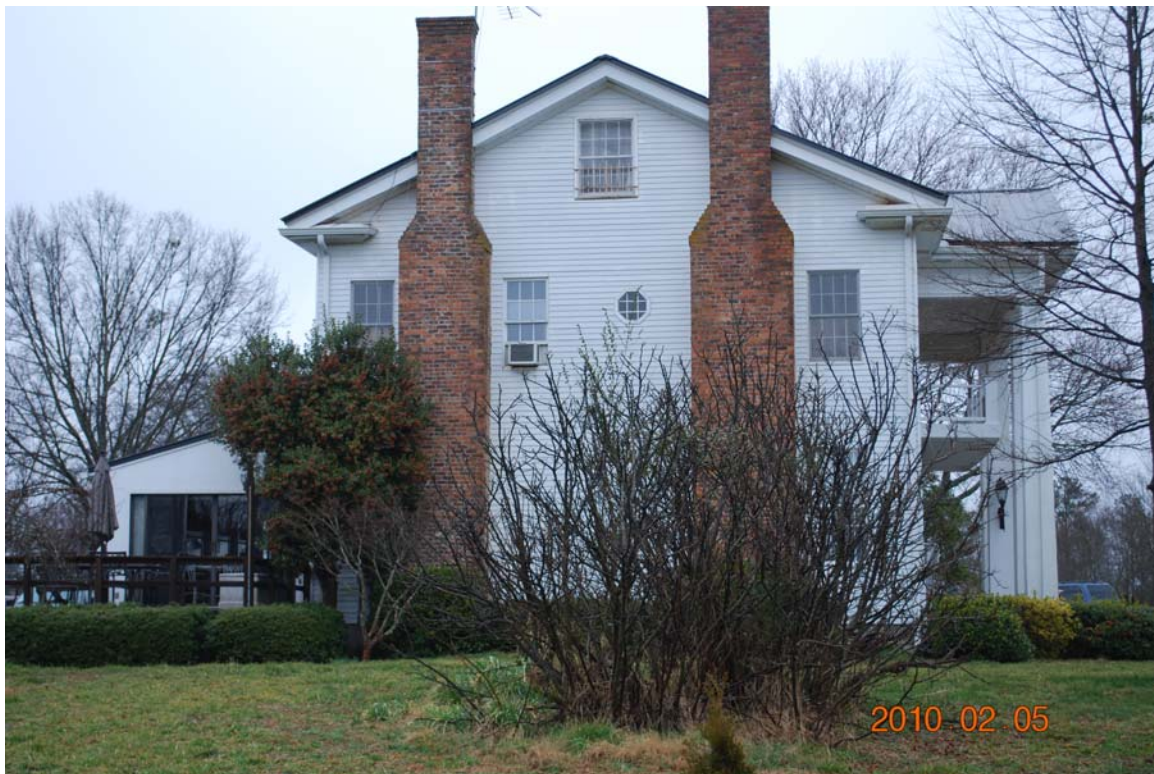
1D: Northerly View of South Facade of Main House
