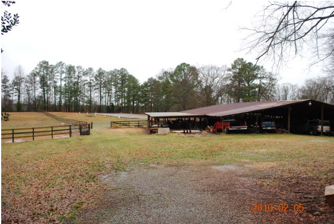
3B: Northwesterly View Toward Open Shed (ECA Structure 3) and Horse Pasture/Ring
