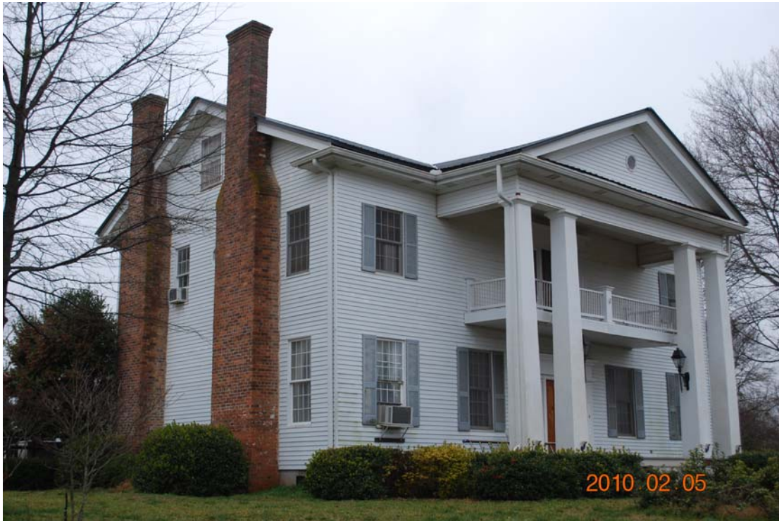
1C: Northwesterly View of Main House
