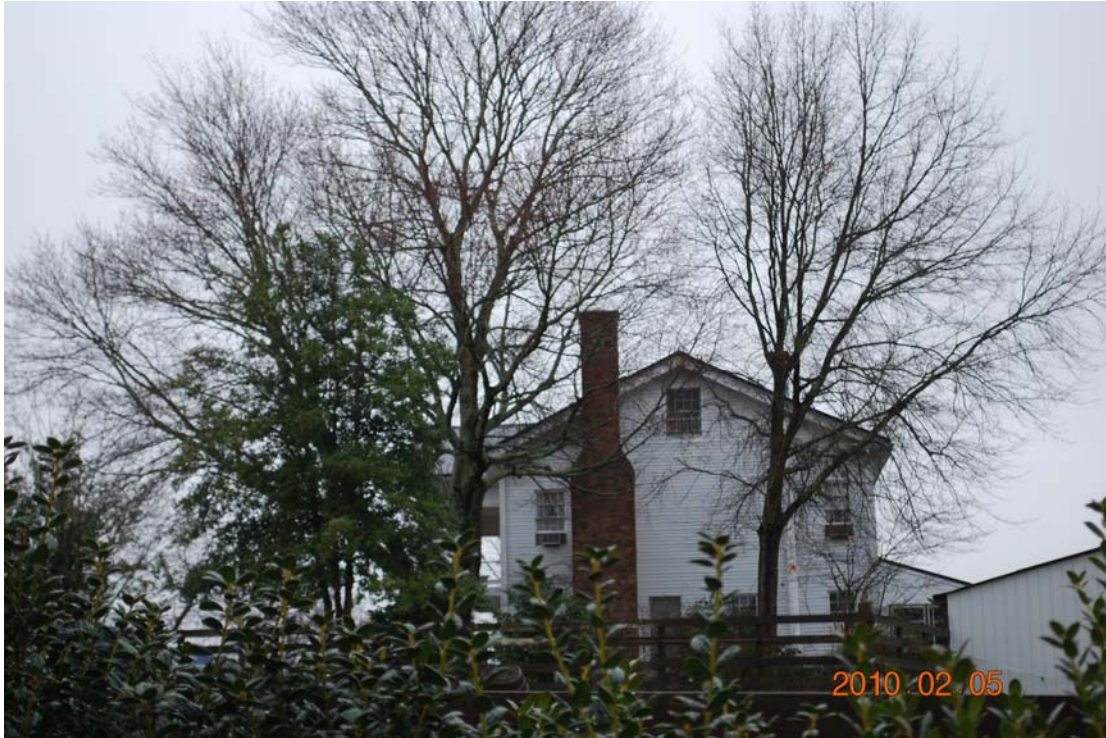
1G: Southerly View of North Facade of Main House
