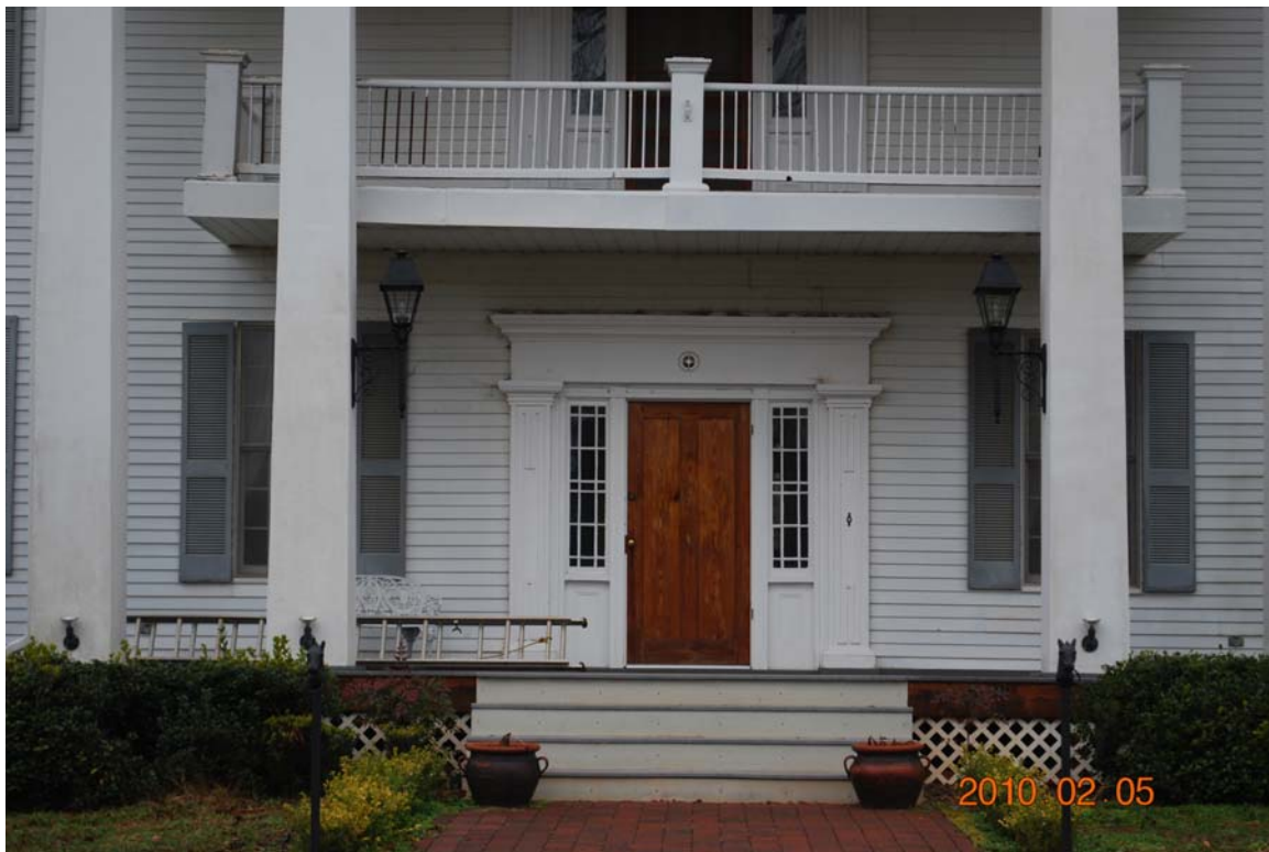
1H: Front Facade and Porch Detailing
