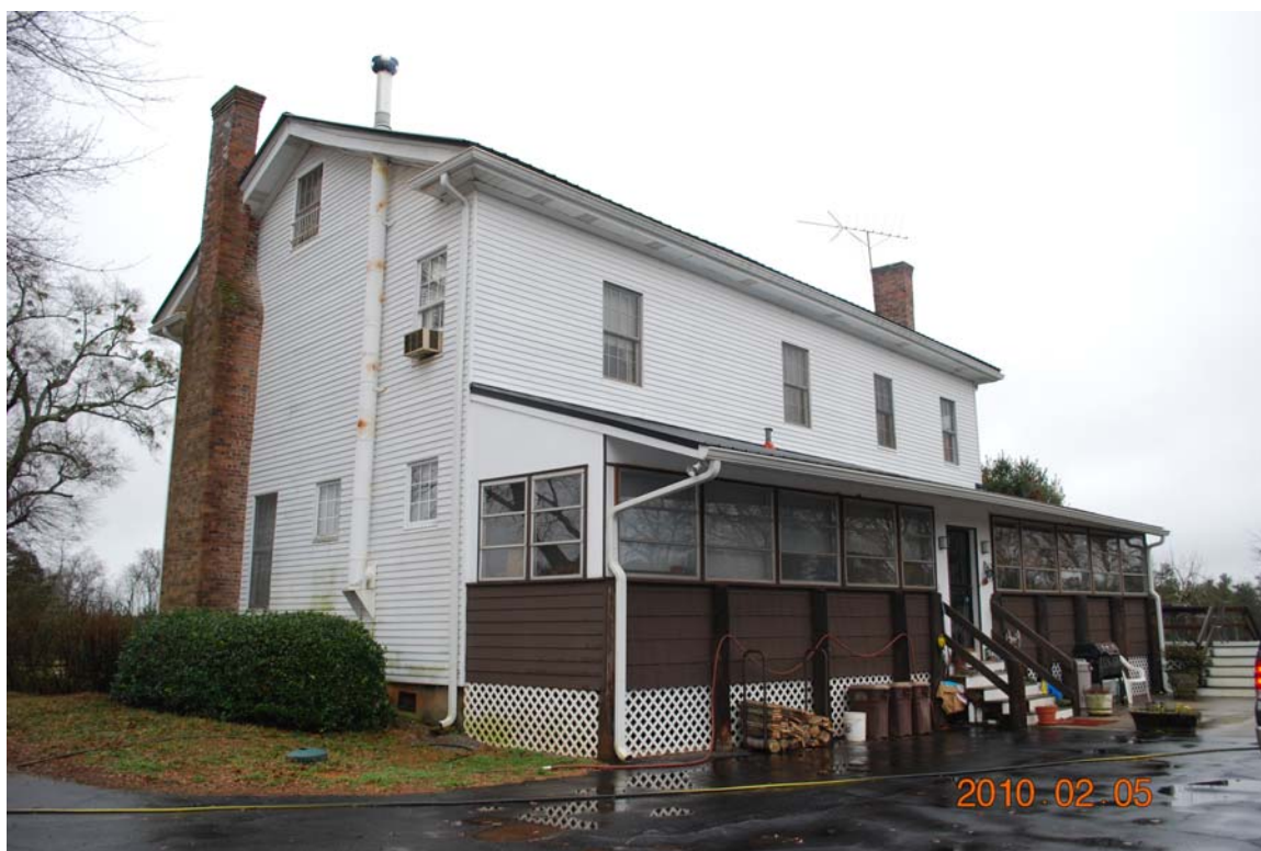
1F: Southeasterly View of Northwest Oblique of Main House
